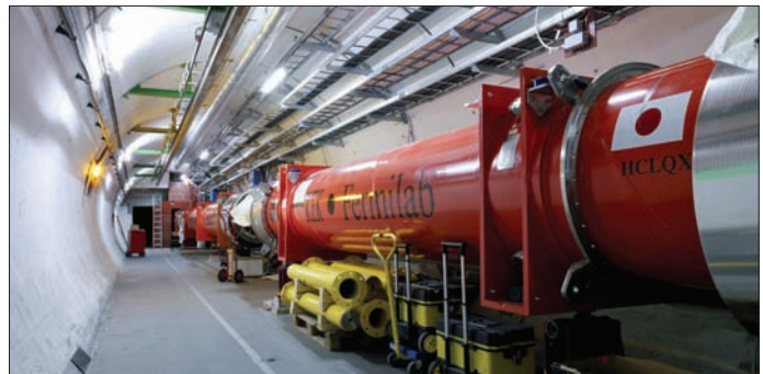
Fig. 1. The interaction-region quadrupole (IRQ) magnet integrated into the BELLE detector and its solenoid magnet at KEKB, top. Fig. 2. The IRQ magnet system installed in the LHC accelerator, bottom.
